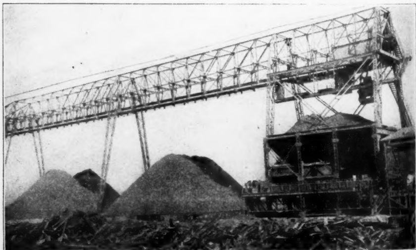
Two Views of the Outside Storage and Reclaiming System
